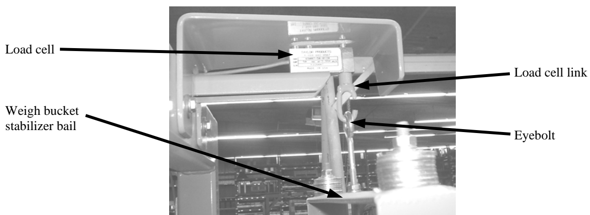
Figure 3-1. Hanging the Weigh Bucket Assembly From the Load Cell
